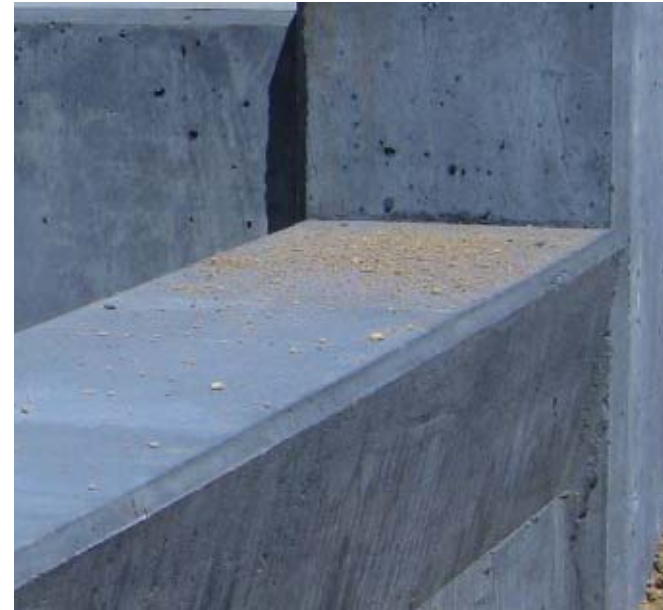
INTEGRAL COLOR CONCRETE WALL
